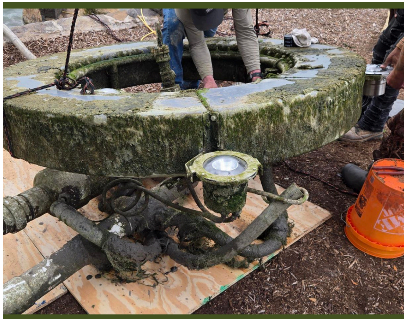
FOUNTAIN LIGHT REPAIRS
