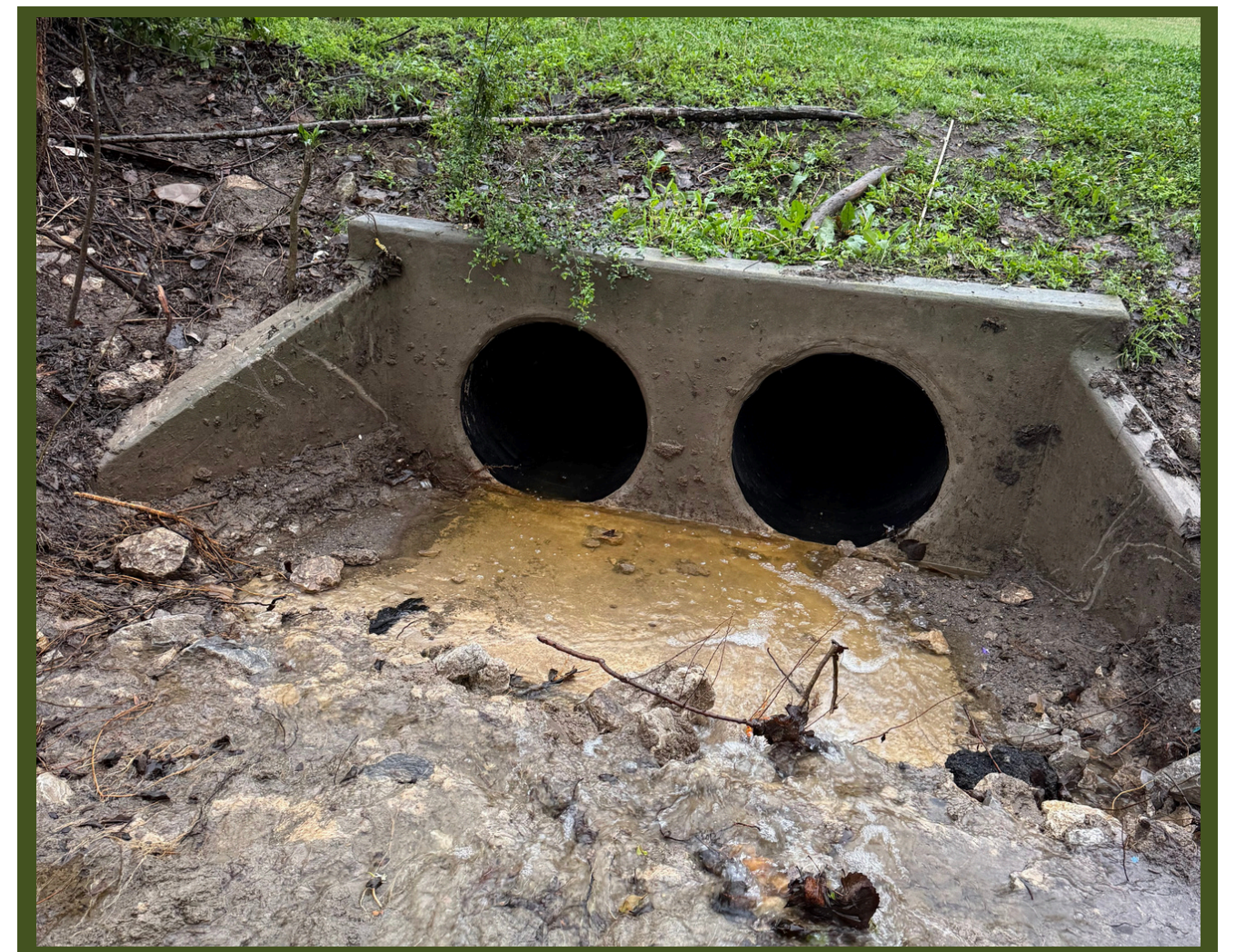
EVA PLACE DRAINAGE WORK
